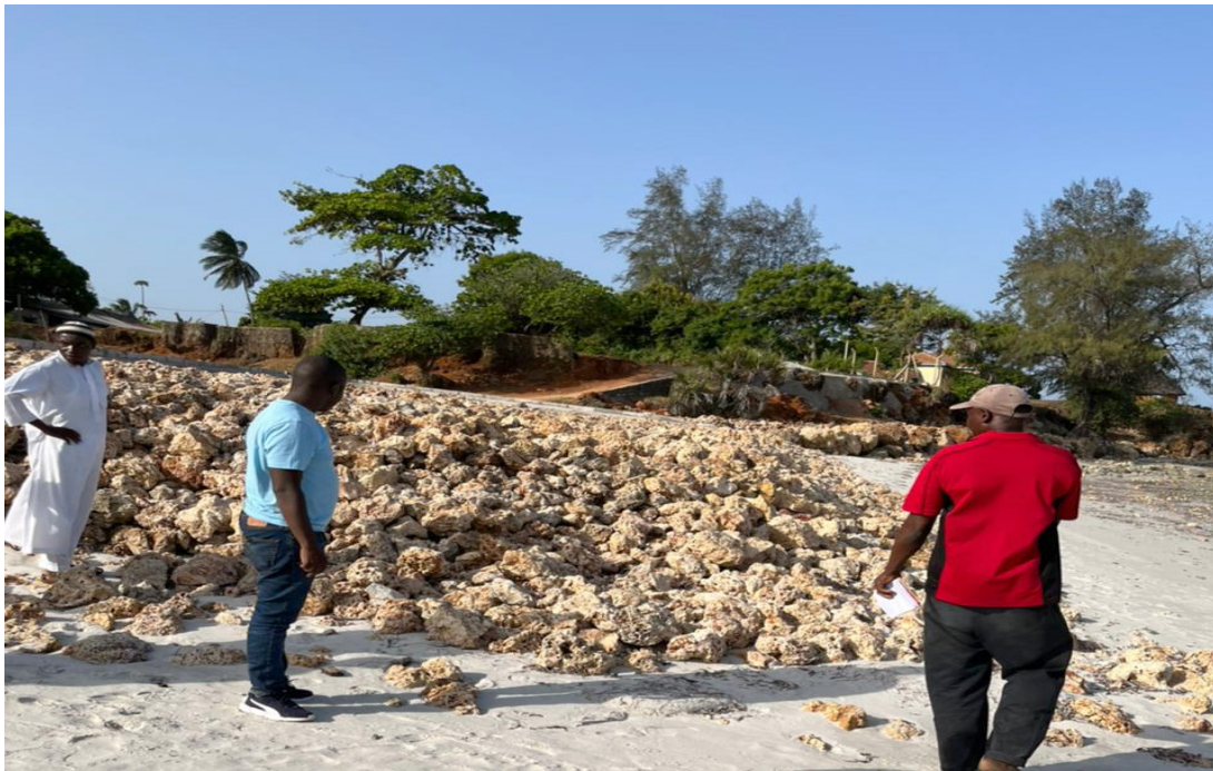
Plate 1: Part of the shoreline stabilisation wall constructed in Mwaembe beach
